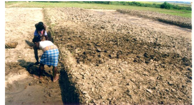
Construction of alternate raised and sunken beds in canal command
