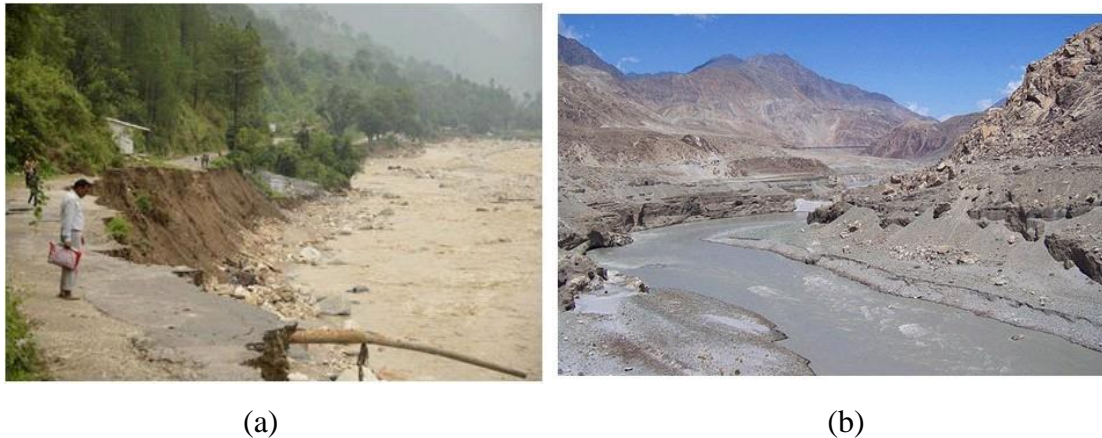
Fig. 2.8 Stream Bank Erosion
